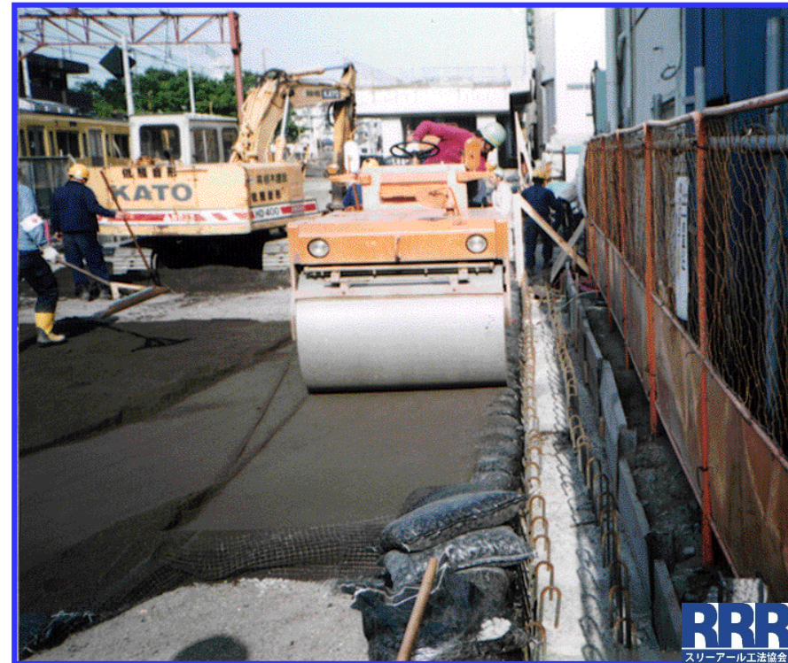
2) Placing geosynthetic & gravel gabions
