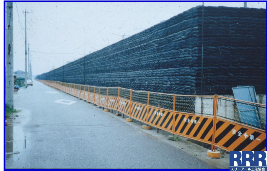
2) Placing geosynthetic & gravel gabions
