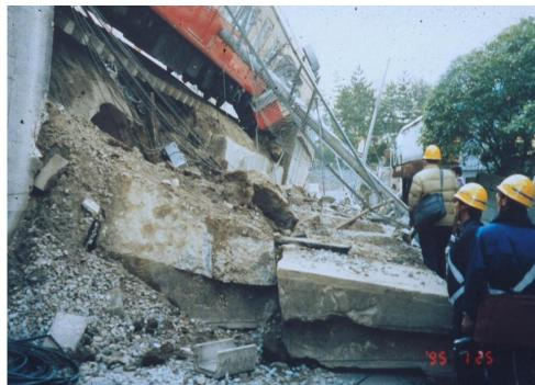
Overturning failure, in spite of seismic design using  $k_h = 0.2$  with  $(F_s)_{allowable} = 1.5$ .
