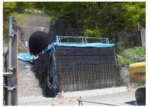
GRS Abutment (before the construction of FHR facing) GRS Integral Bridge at Haipe, Sanriku Railway (total span length= 60 m)
