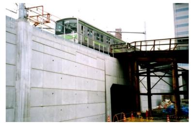
"The use of: 1) dense geogrid layers; 2) several long geogrid layers; and 3) FHR facing" enhances monolithic behaviour of the enlarged reinforced zone without developing local internal failure!
