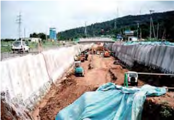
Nail-reinforced soil wall under construction, Kyushu Shinkansen, 2000
