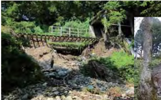
Collapsed railway embankment by Niigata and Fukushima torrential rains of July 2011
