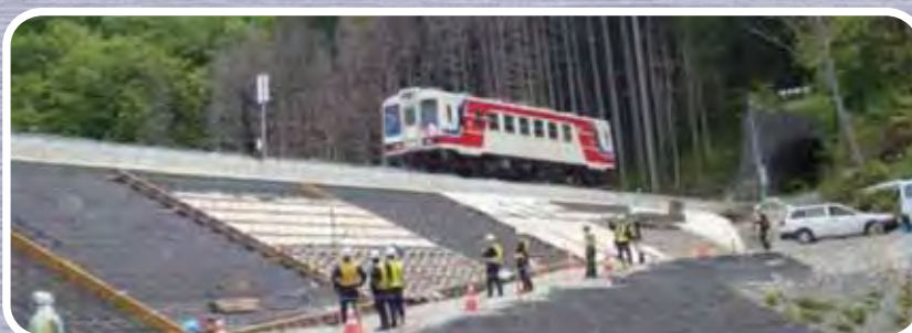
GRS structure to prevent water-front disasters, Sanriku Railway, Tanohata, 2015
