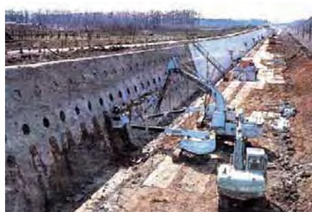
Nail-reinforced soil wall under construction, Tohoku Shinkansen, 2000
