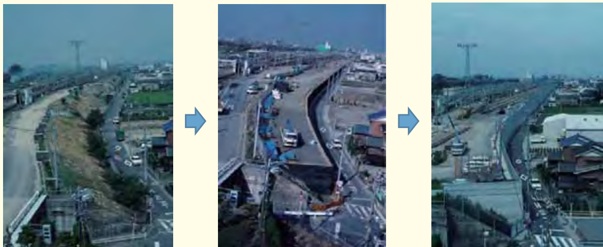
Shinkansen yard at Biwajima, Nagoya, 1989 - 1990 ( average wall height= 5m & total length= 930m)
