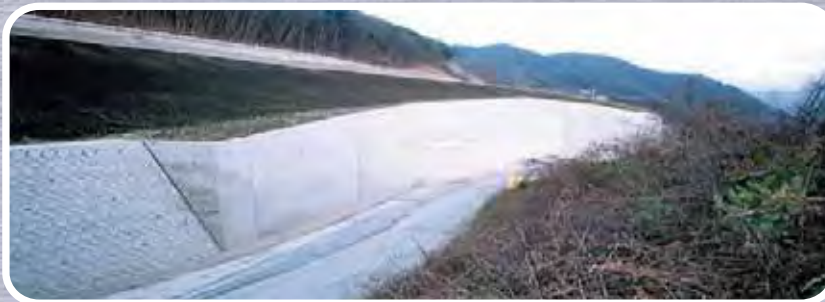
GRS retaining wall, Yamagata Expressway, 1997
