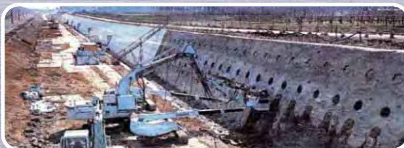
NRS retaining wall, Tohoku Sinkansen, Morikoka, 2000
