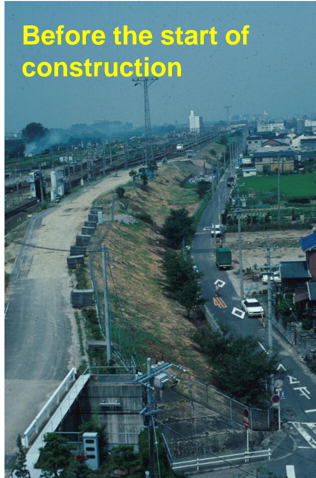
Completed GRS wall, but before the construction of FHR facing
