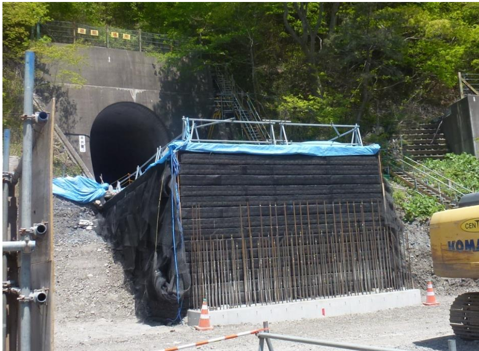
GRS Abutment (before the construction of FHR facing)
