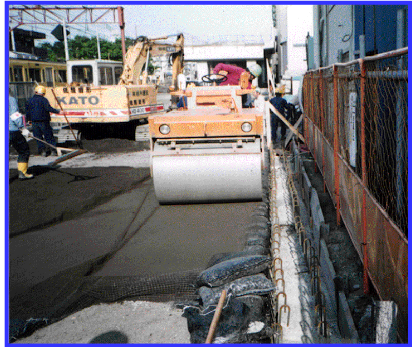
2) Placing gravel bags wrapped-around with geogrid
