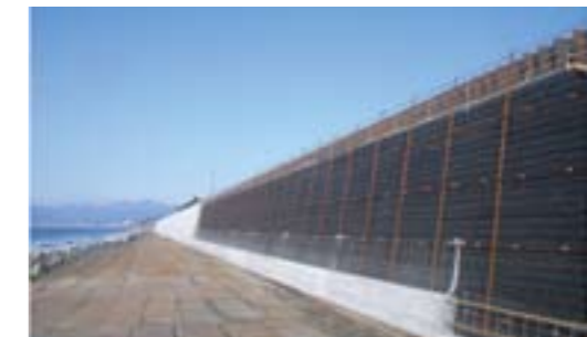
壁面工の建設前後 Before and after the construction of facing.
