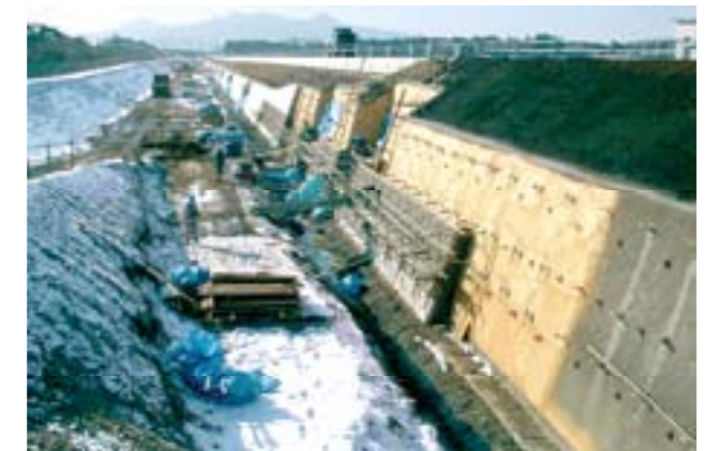
Nail-reinforced soil wall under construction (for Tohoku Line of high speed train) 既設のり面急勾配化工法の事例(東北新幹線)
