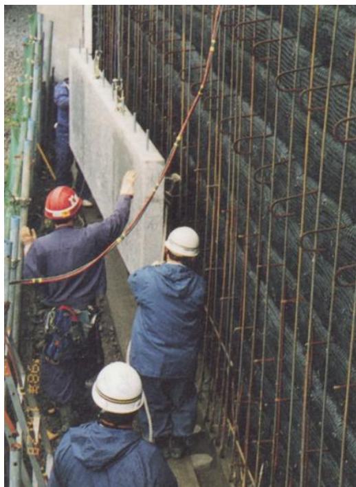
Photo 3.2.8-4 Installation of RRR-panel
