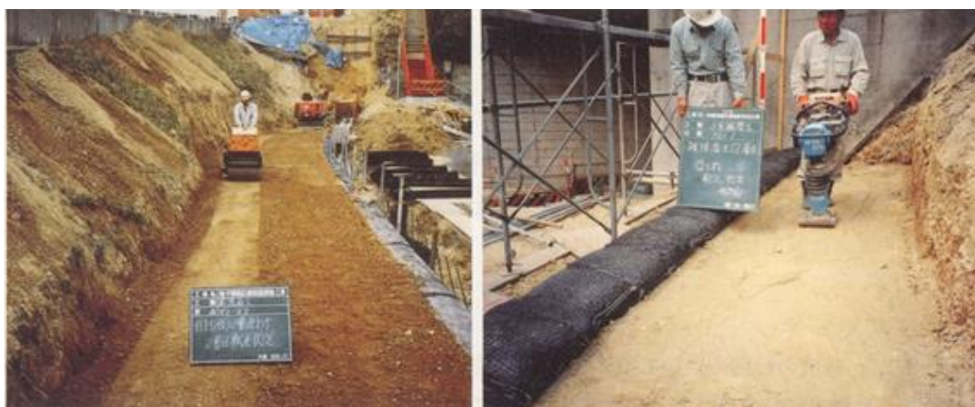
Photo 3.2.7-1 Compaction of backfill soil by manpower
