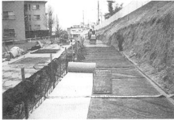
Photo 3.2.2-1 Installation of drain blanket on the base ground
