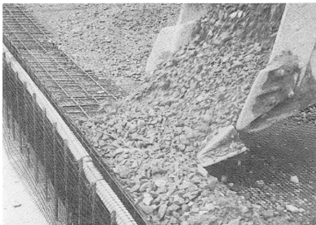
Photo 3.2.6-6 Throwing of crusher run
