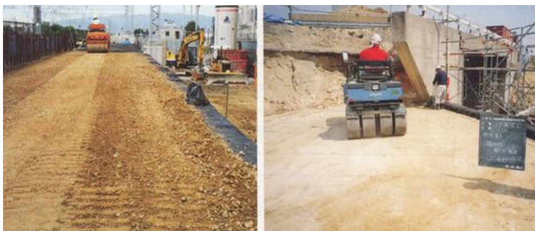
Photo 3.2.7-2 Compaction of backfill soil by heavy compactor
