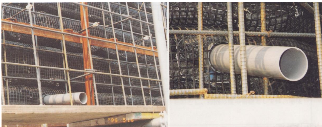
Photo 3.2.9 Installation of drain pipes
