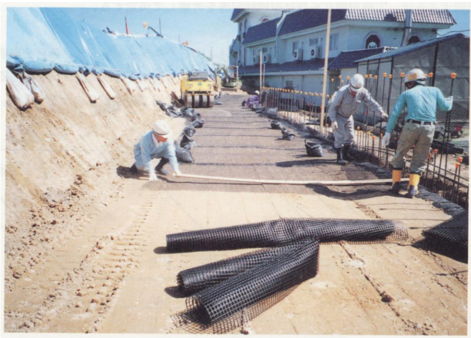
Photo3.2.5-1 Installation of geosynthetic
